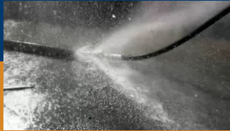
PIPE DESCALE & REBORE
